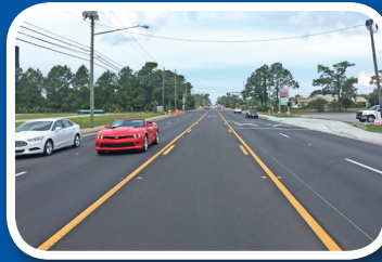
@ S.R. 77 (Martin L. King, Jr. Boulevard) Intersection
