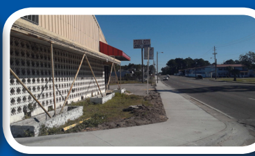
@ S.R. 77 (Martin L. King, Jr. Boulevard) Intersection
