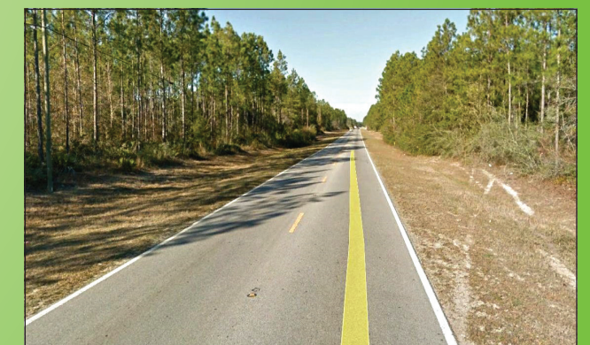
Existing C.R. 2315 (Star Avenue)
