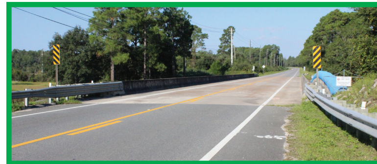
Burnt Mill Creek Bridge location.
