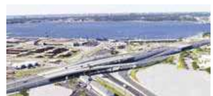
Completed flyover of the elevated U.S. 98 over 23rd Street in Panama City, Fla.
